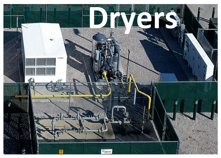
Dryers are used to reduce the moisture content and filter the gas before it enters the compressors. Removing water vapor can reduce the risk of corrosion and blockage in the fuel compression systems and vehicles. Dryers are customized for each customer's specific requirements.
